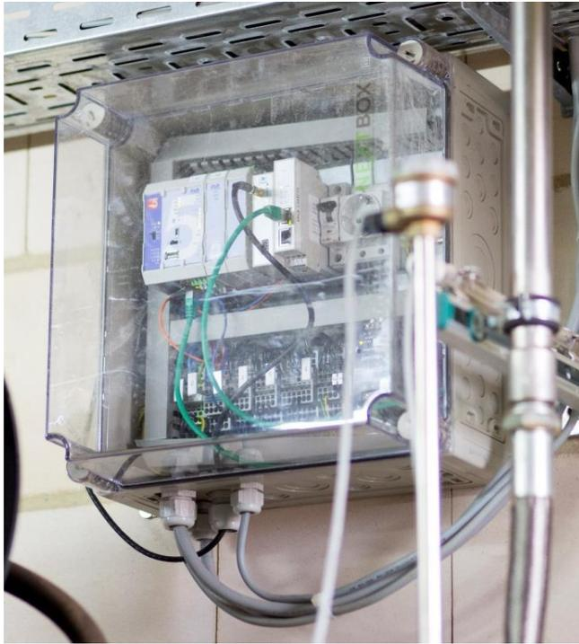
The Next Box is individually configured for the type of unit: district heating, gas or water storage, and any timetable restrictions are programmed, so the unit can always operate under optimal conditions, technically and economically.
